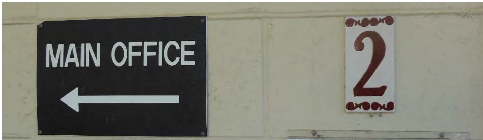
S1. Exterior room identification and wayfinding signs; non-compliant.
