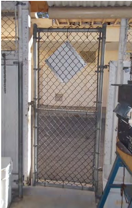
D3. Classroom patio; locked gate to exterior.
