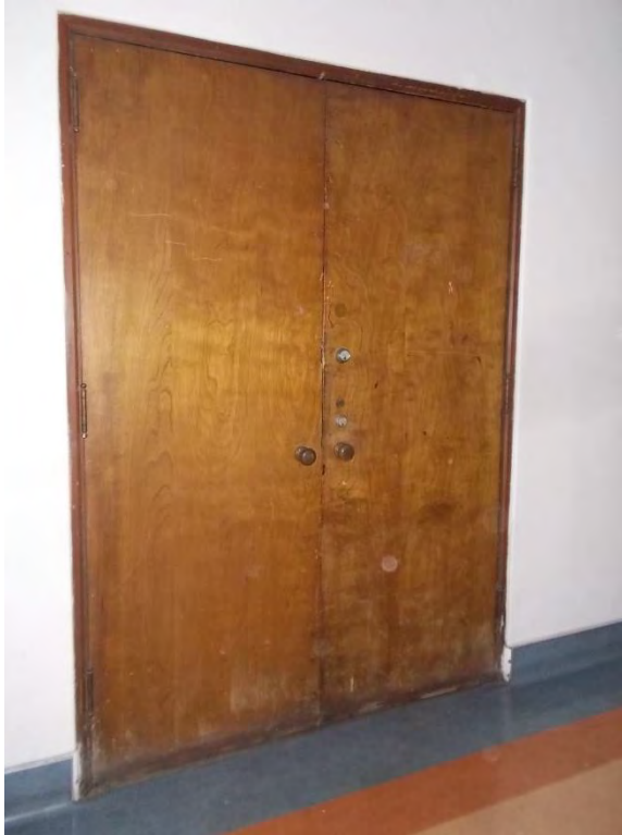
D1. Second floor equipment room doors.
