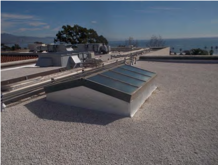
R1. Skylight at built-up roof system, in good to excellent condition.
