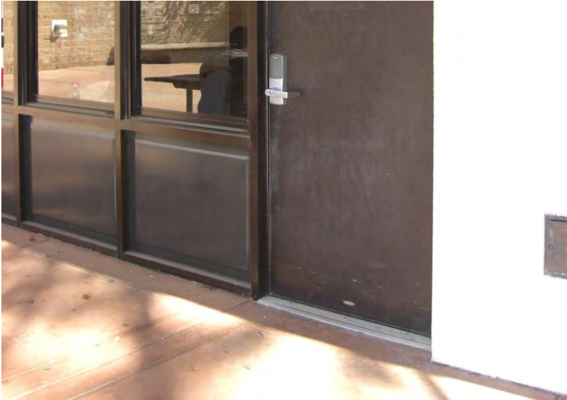
EF1. Second floor exterior colored, scored concrete walkway; good condition.
