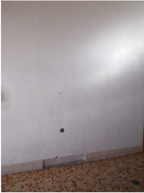
A13. First floor Men's Restroom.
