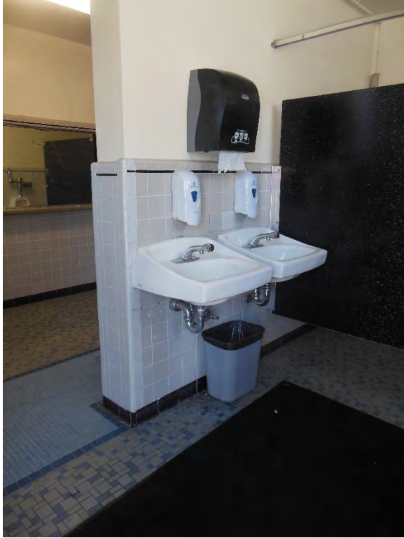
RR3. Men's Restroom; lavatories and fixtures.
