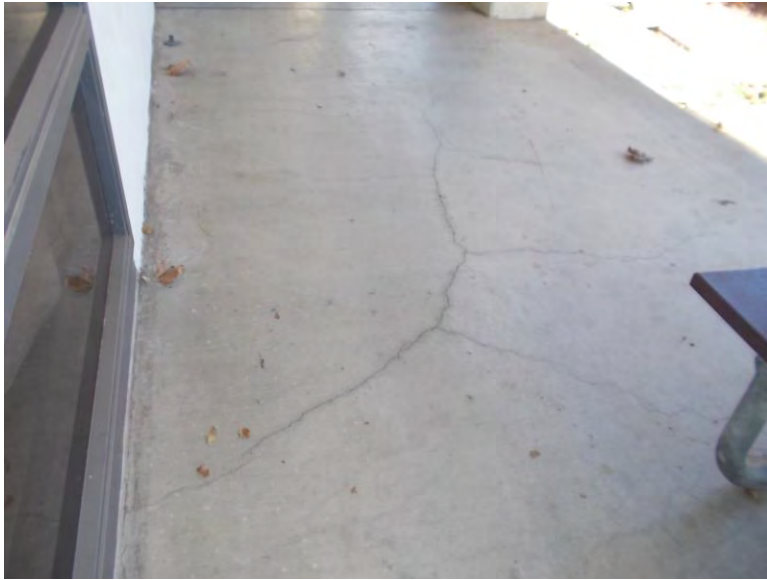
EF3. Southeast OE exterior corridor.
