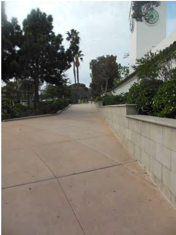
PT2. West side of building; excessive cross and longitudinal slopes along path of travel.
