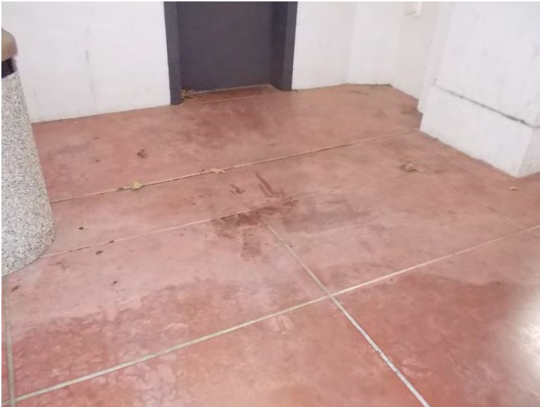
EF2. Northwest entrance to Elevator.
