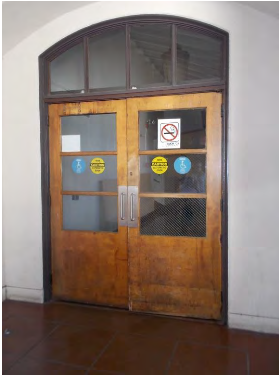
D1. First Floor entrance doors near elevator.
