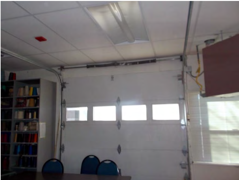
D2. Classroom 32; interior roll-up door.
