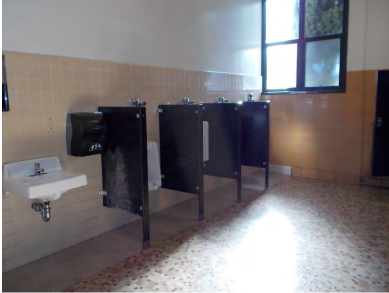
RR3. Mens restroom, first floor southwest wing.
