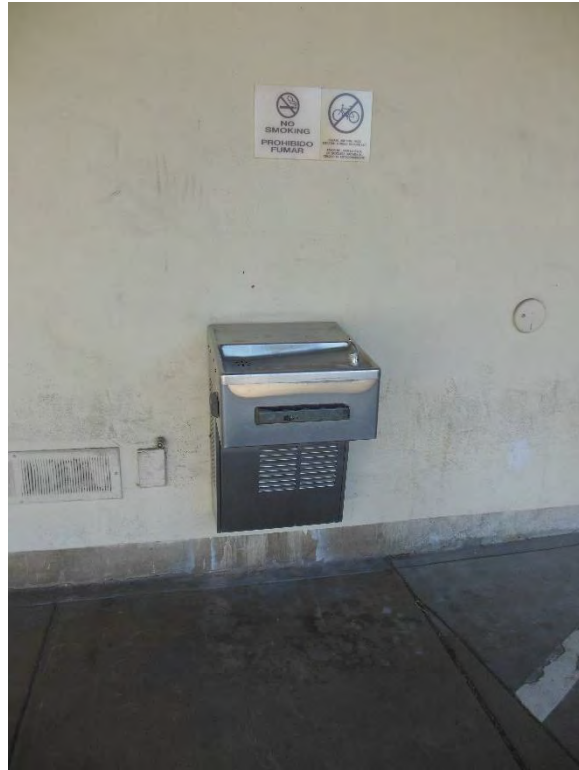
DF2. Drinking fountain in exterior walkway; Handrails not provided.
