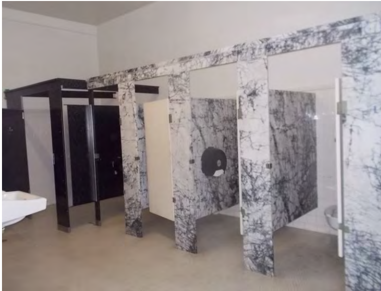
RR3. Women's Restroom; toilet compartments.
