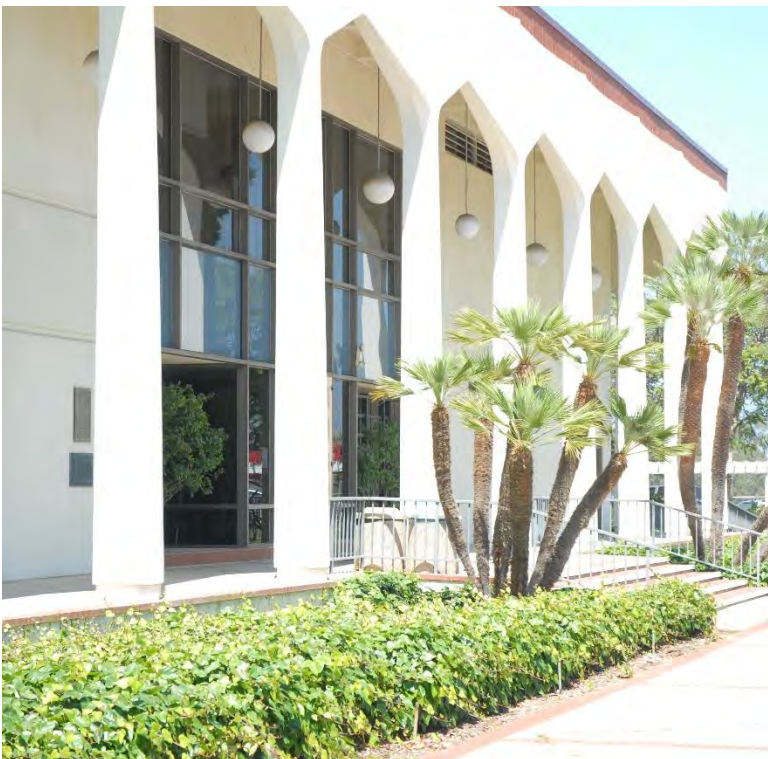
EW2. Exterior storefront; east side.
