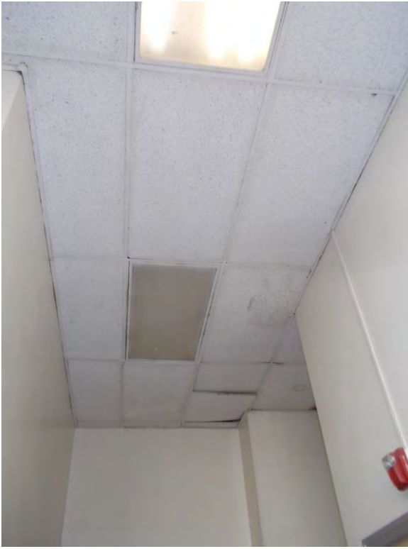
C3. OE second floor corridor.
