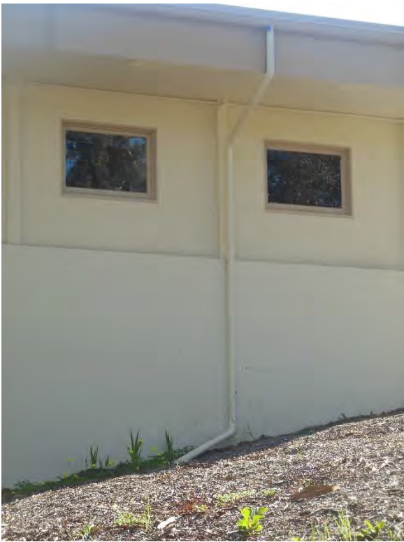
AE4. Exterior painted concrete and plaster.
