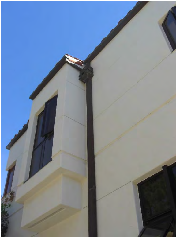
R4. Clay tile roof system with metal downspouts, in good condition.
