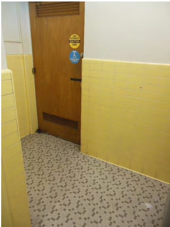
AI4. Restroom foyer, original ceramic tile wainscot.
