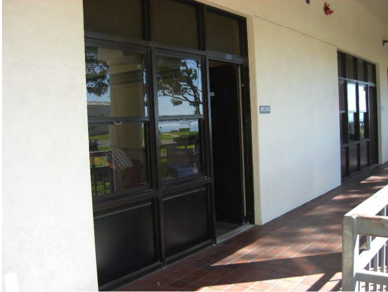
EW1. West wall, second floor storefront window system in good condition.
