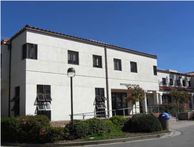
AE1. West facing entrance plaster wall.
