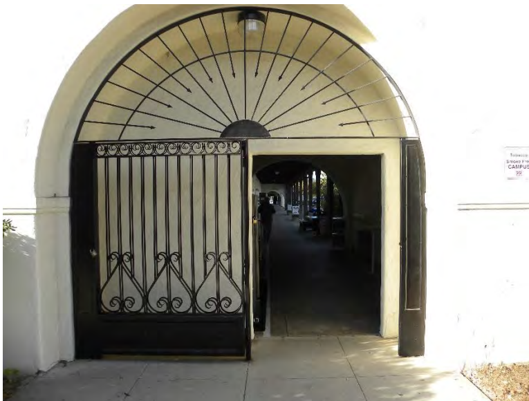
D2. Entrance from east side of site; missing ISA signage.
