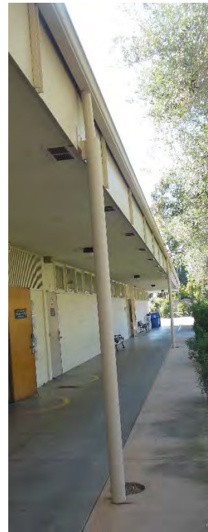
R2. Gutter and downspout.
