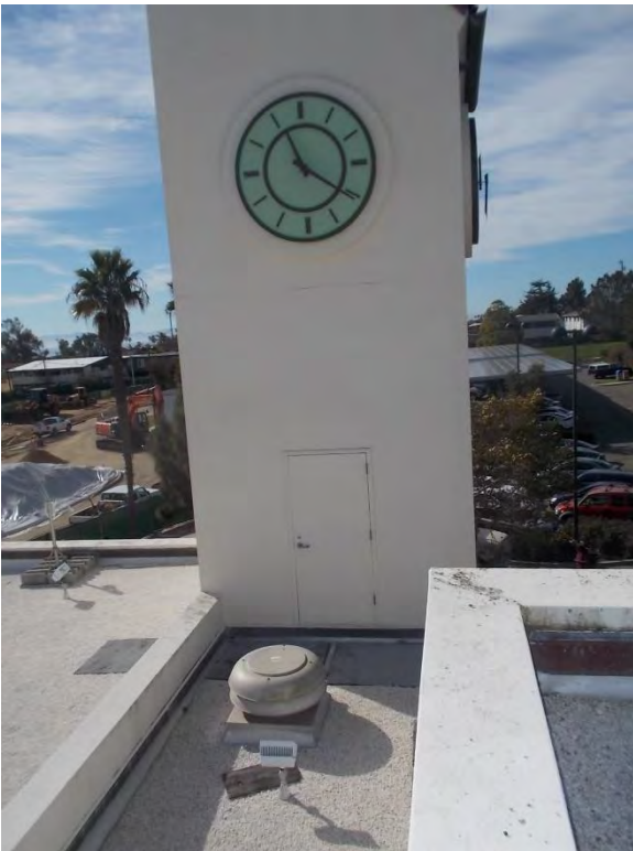
R4. Clock tower at plaster parapet.
