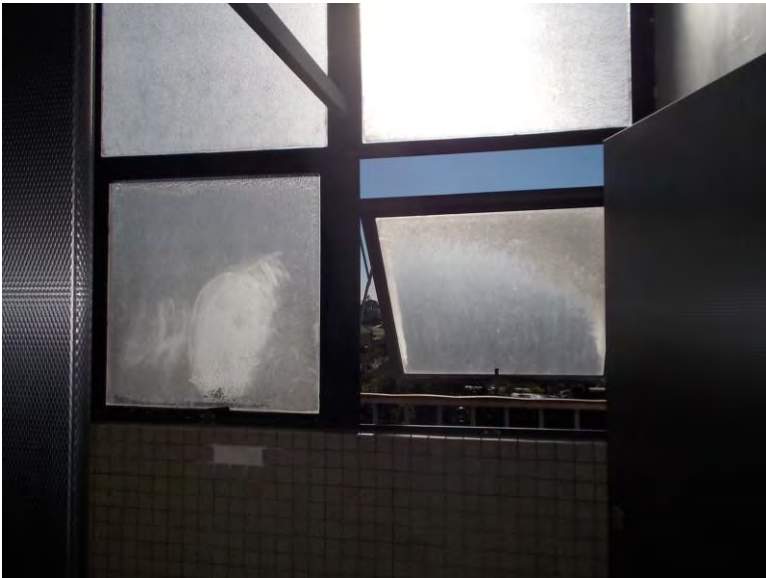
EW5. Second floor Women's restroom.
