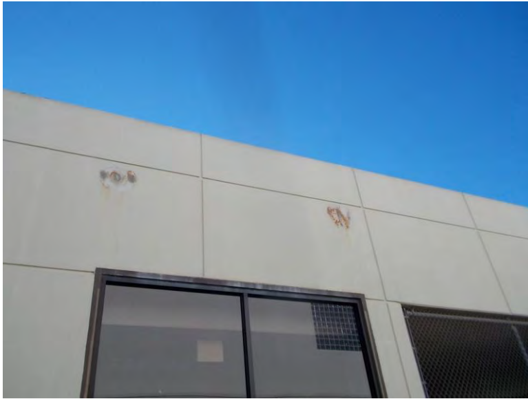
AE5. OE building, exterior wall facing Auto Quad.
