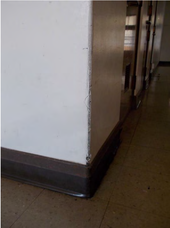
AI1. Interior corridor corner.
