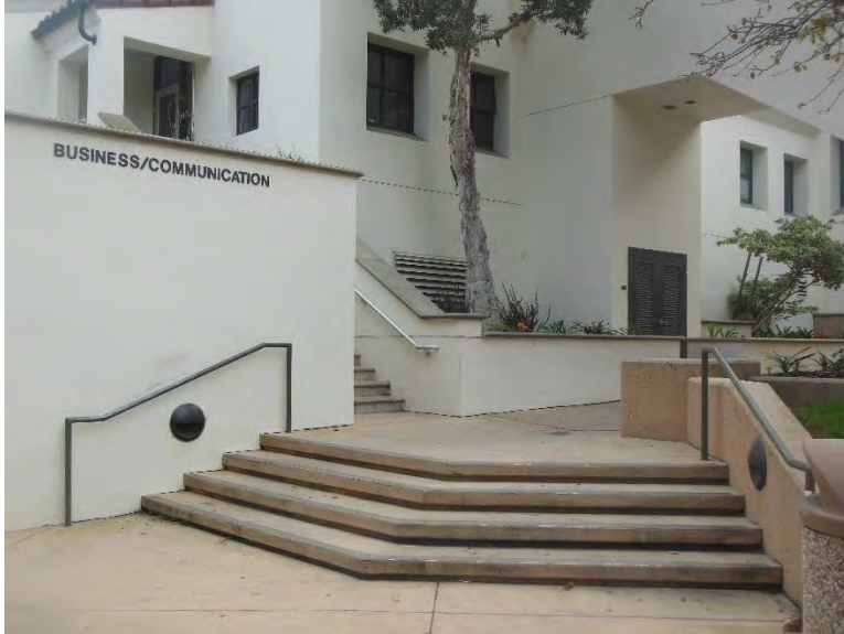
PT6. East side of building; non-accessible entry lacks wayfinding signs directing user to ramped entry location.
