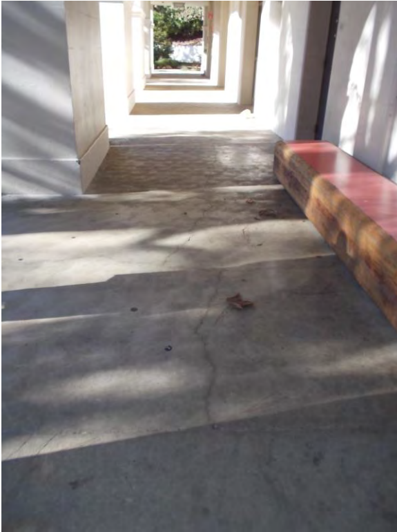
EF1. Northwest exterior corridor.
