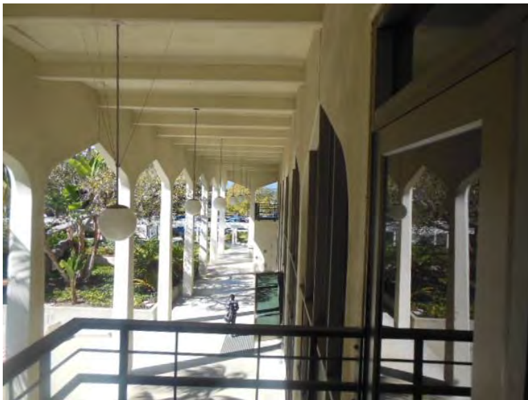
R2. Exterior underside of roof overhang.
