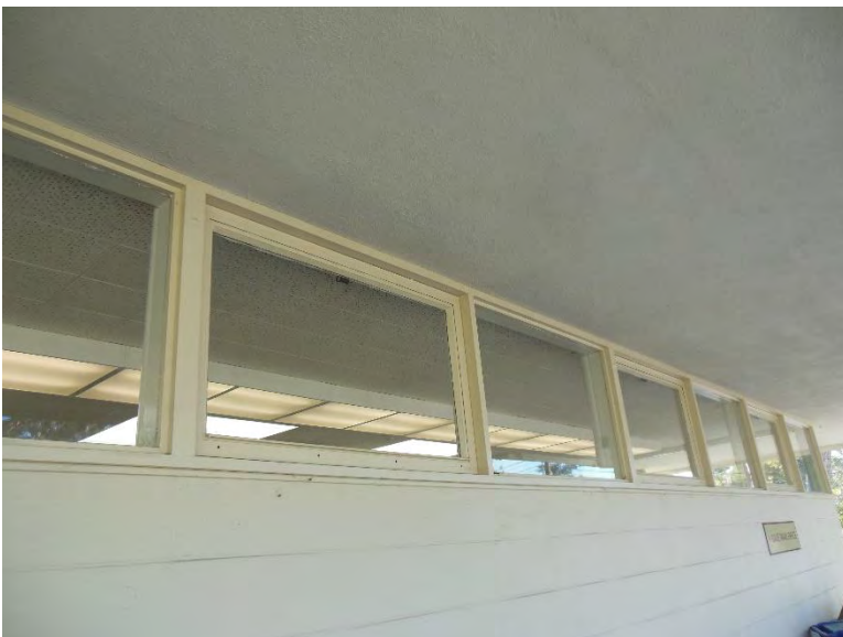
EW2. Exterior fixed wood windows; new paint.
