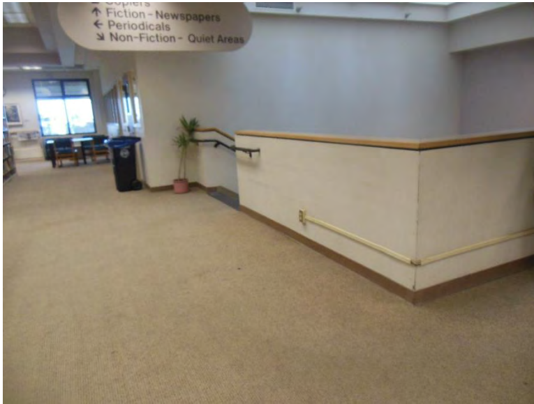
ST1. Library main interior staircase; ADA signage missing.
