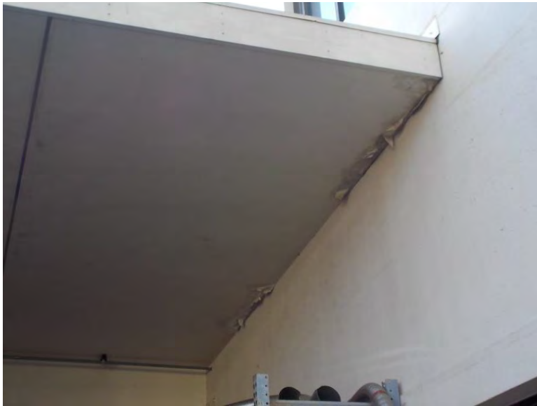
AE6. OE building, southeast exterior overhang.
