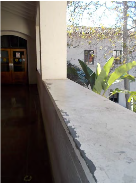
AE4. Northwest exterior walkway wall.
