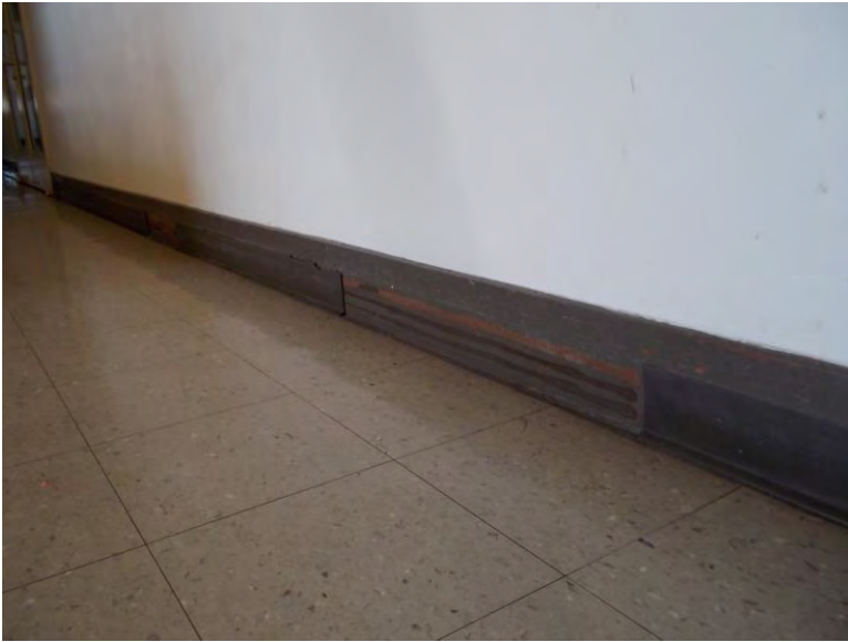
IF3. Southwest corridor second floor.
