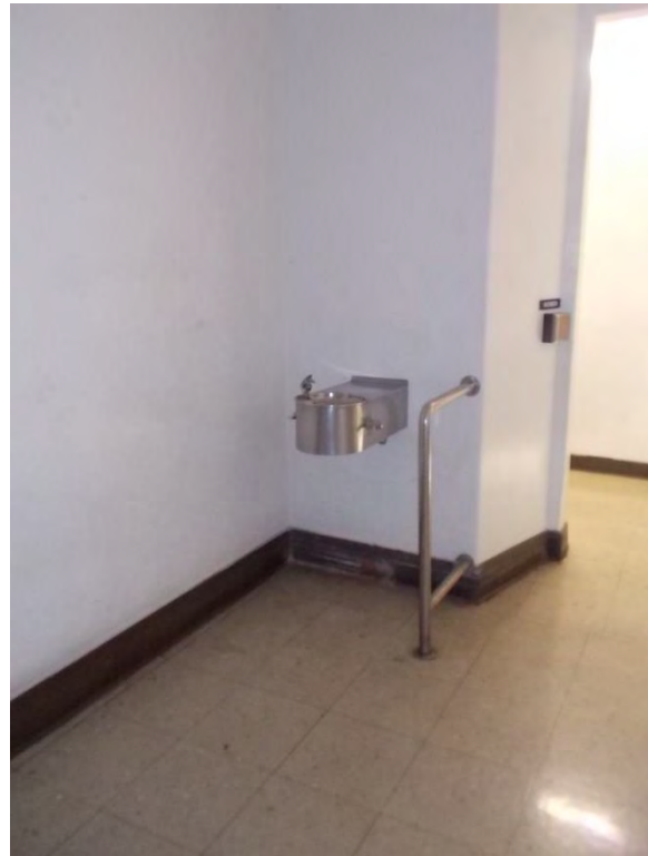
DF1. Second floor drinking fountain at restrooms.
