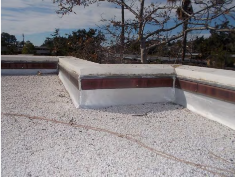
R3. Built up roof with plaster parapet.
