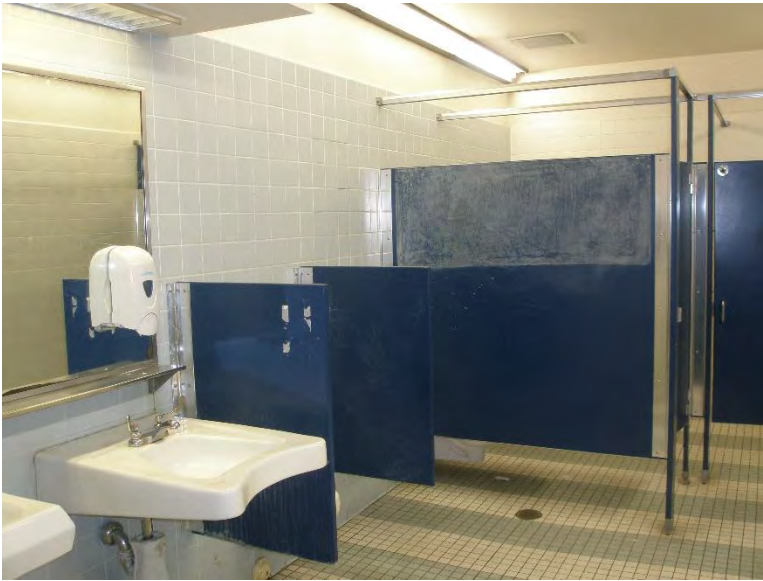
RR1. Mens restroom, accessible clear floor space not provided. Mirror and soap dispenser mounted above ADA compliant heights.
