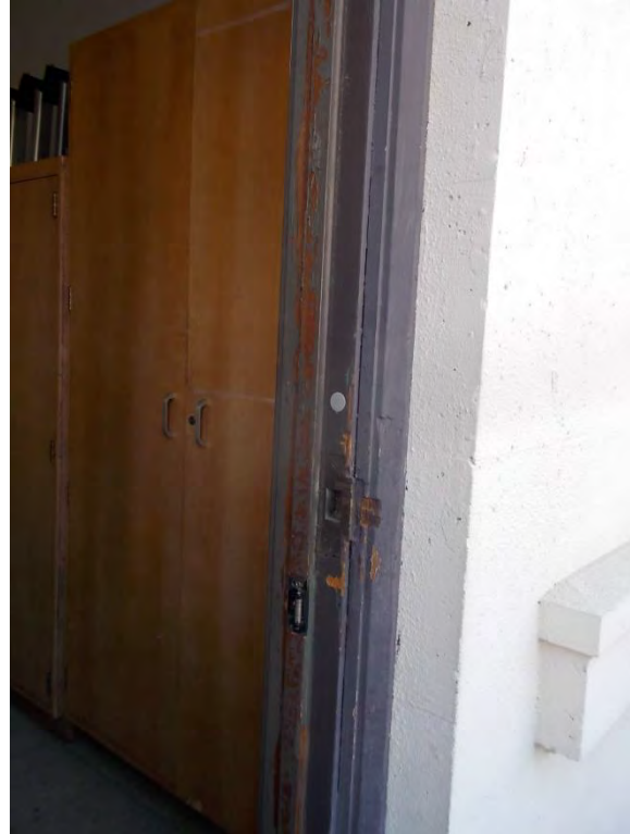
D2. 2nd floor exit door to stairs.
