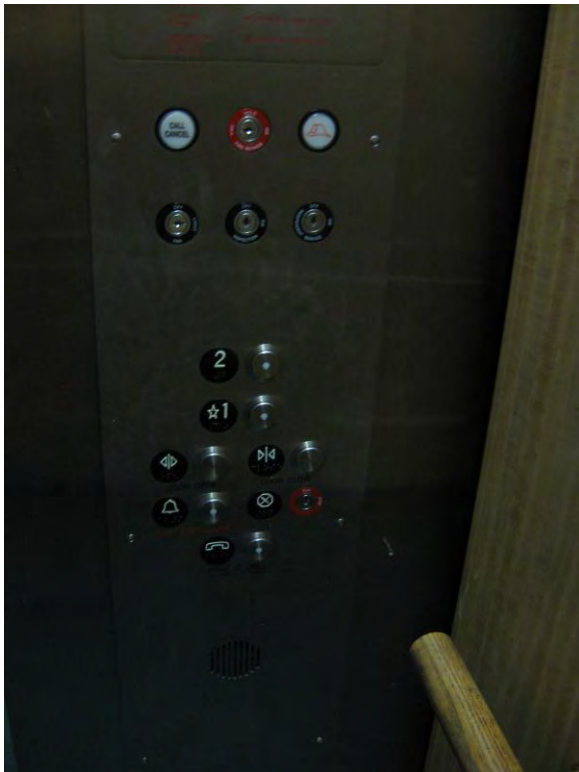
EV2. Elevator car interior.
