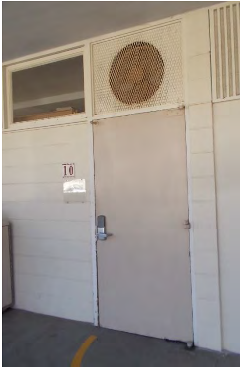
D1. Classroom 16; exterior door; fan in transom.
