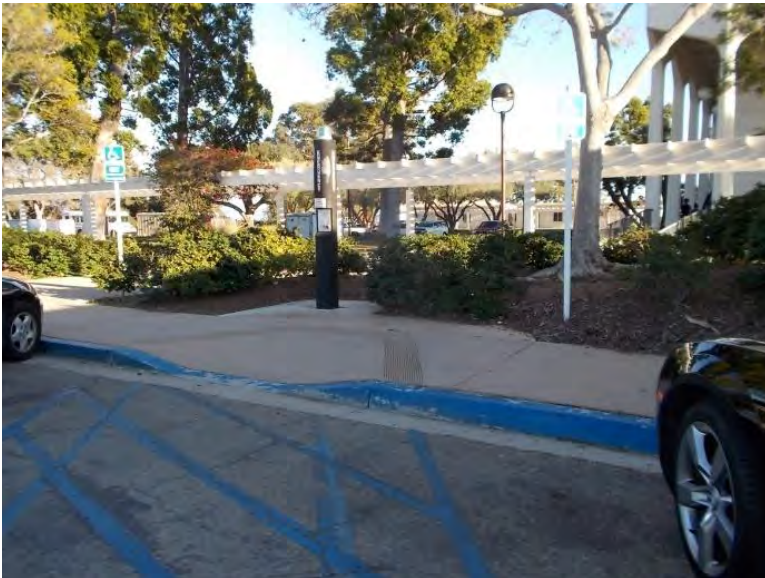
PT4. Non-compliant curb ramp. Truncated domes are not present, and top landing is not deep enough. The emergency phone also impedes into the clear space of the upper landing. Accessible parking stall stripping is faded and markings unclear.
