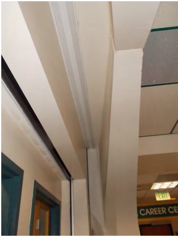
C1. Second floor Atrium infill space; building expansion joint cover.
