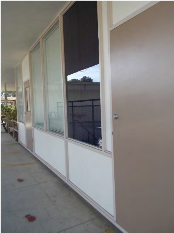
EW1. Exterior fixed wood windows; new paint.
