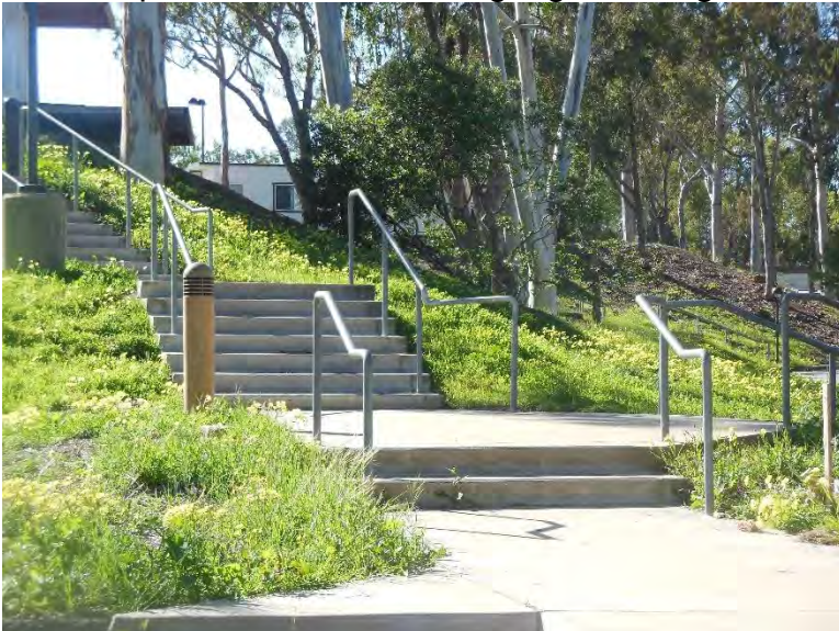
ST2. Exterior stairs from lower lot to upper campus; non-compliant handrails, stair nosing and signage missing.
