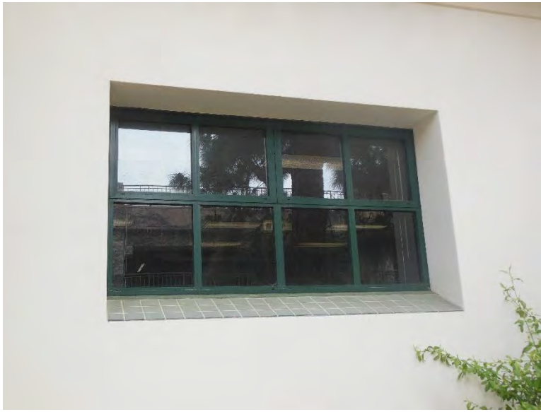
EW1. Aluminum framed lower floor windows and sill in good condition.
