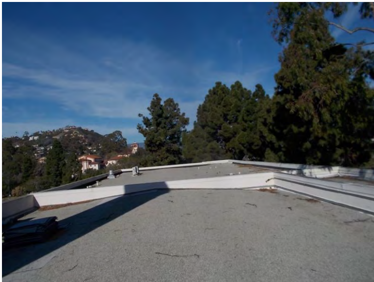
R2. Northeast wing built-up roof.
