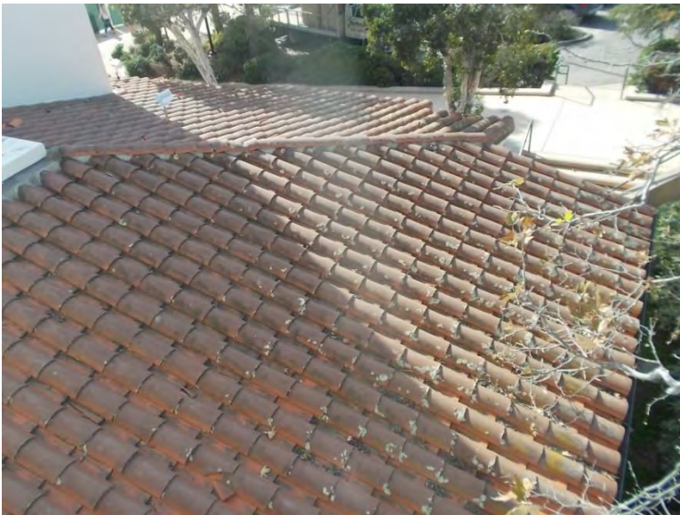
R2. Mission clay original roof tile.
