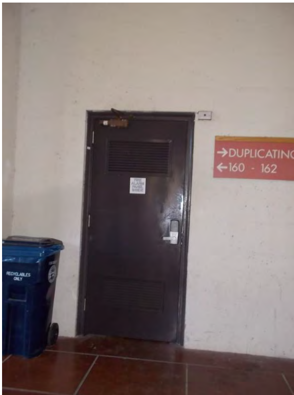
D3. Entry door to 1st floor Duplicating.
