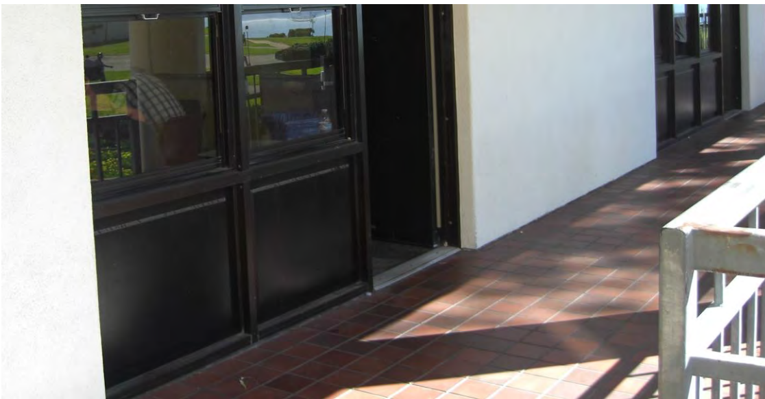
EF2. Second floor exterior ceramic tile walkway; good condition.
