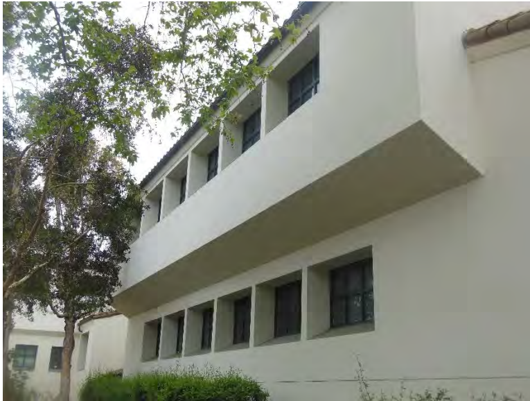
EW2. Aluminum framed lower and upper floor windows in good condition.
