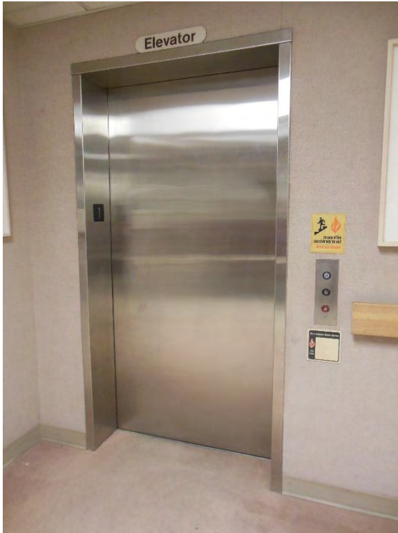
EV1. Library; first floor elevator entrance.
