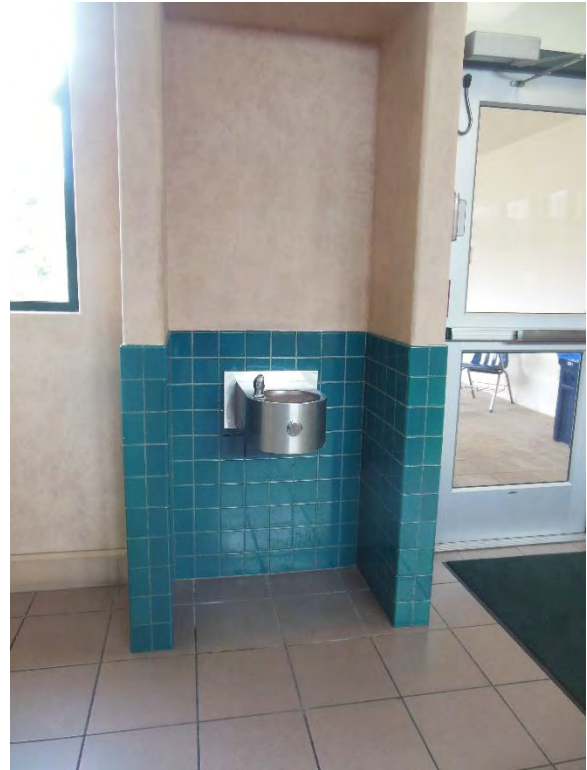
DF2. Third floor; single drinking fountain.
