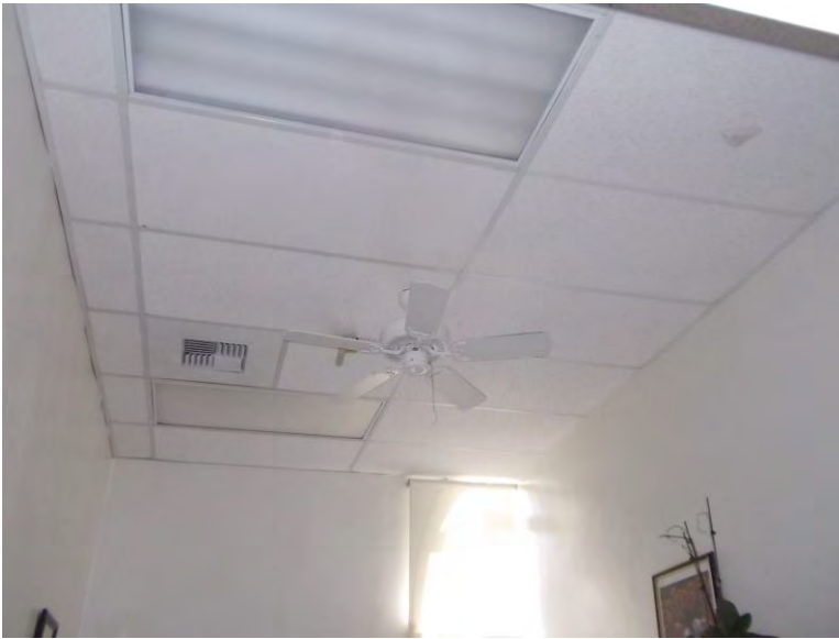
C1. Office; suspended acoustical ceiling system.
