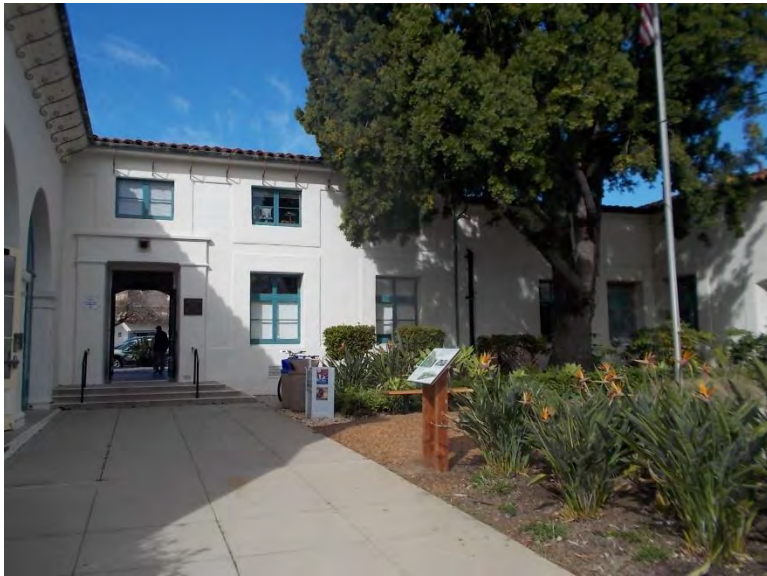
PT1. Exterior walkway to south entry; path of travel with excessive slopes, hazardous surface features, and no wayfinding signage.
