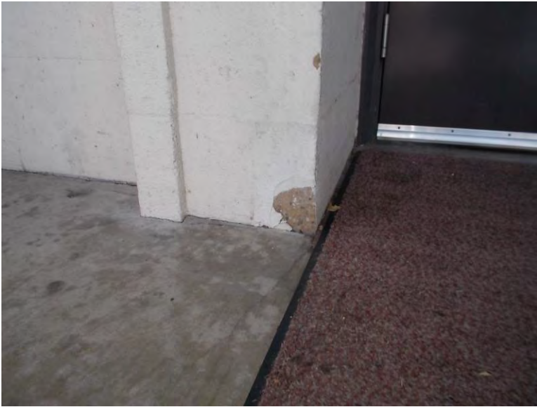
AE3. Northeast exterior entrance column.
