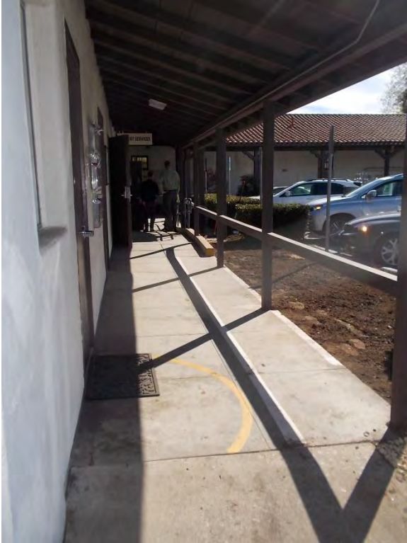
PT7. Exterior walkway; path of travel interrupted door swing, and curb edge not provided.
