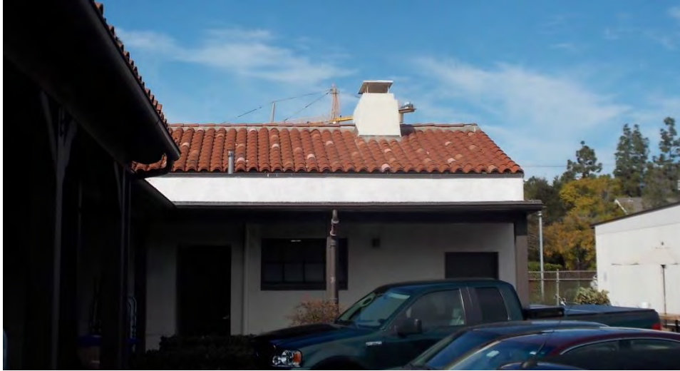
R3. Kitchen; clay tile and roof chimney/vent, and built-up roofing over walkway canopy.
