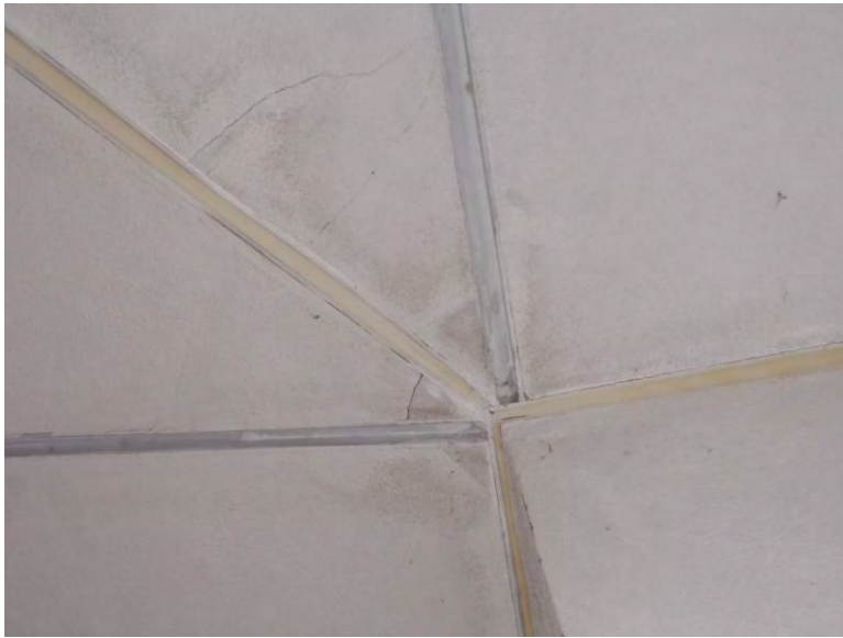
A14. Building joints.
