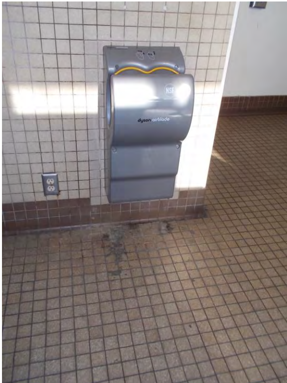
RR4. Womens restroom, second floor southwest wing.
