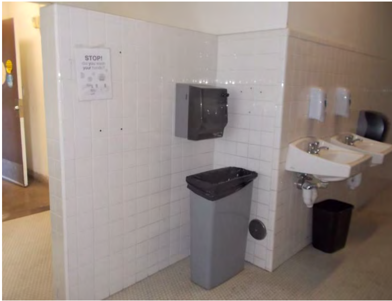
RR1. Women's Restroom; lavatories and fixtures.
