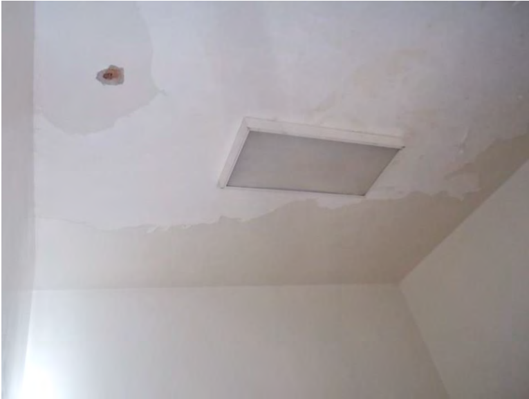
C1. First floor Women's Restroom.
