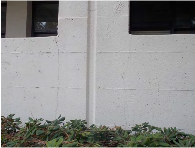
AE1. Northeast exterior walkway wall.
